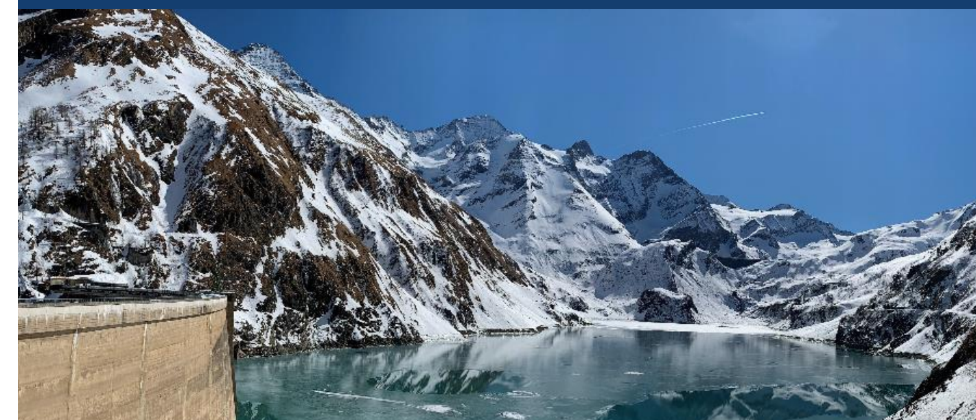
Power Plant Limberg III, AT
