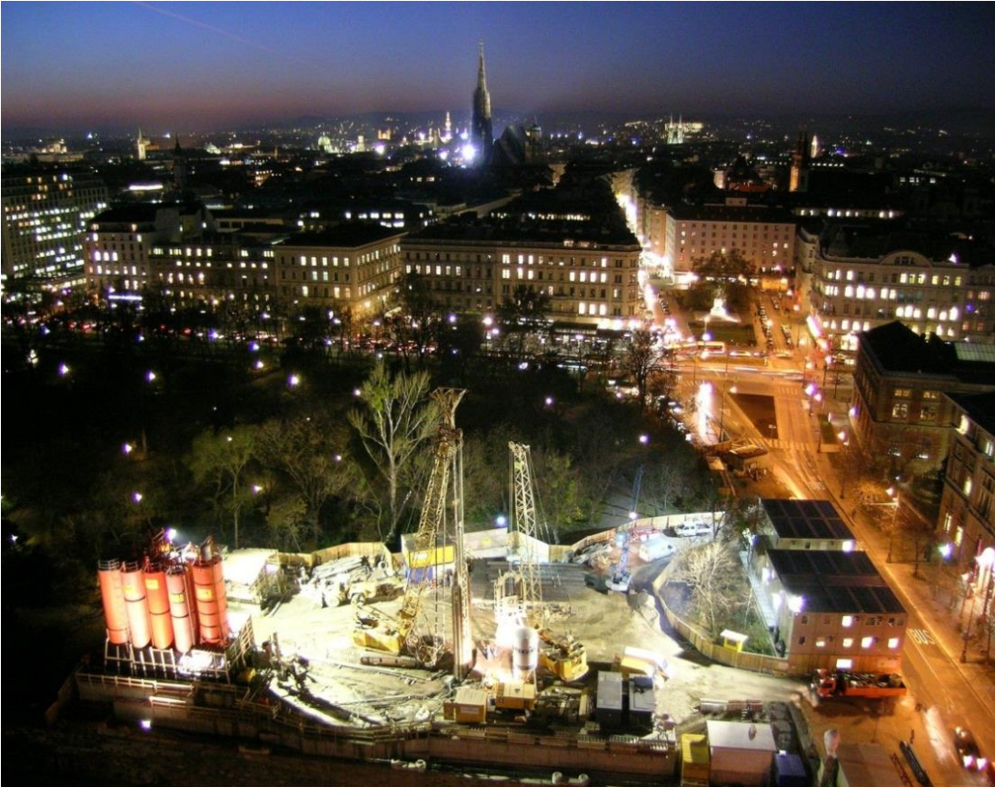
2004: Large scale sewage project, Vienna
