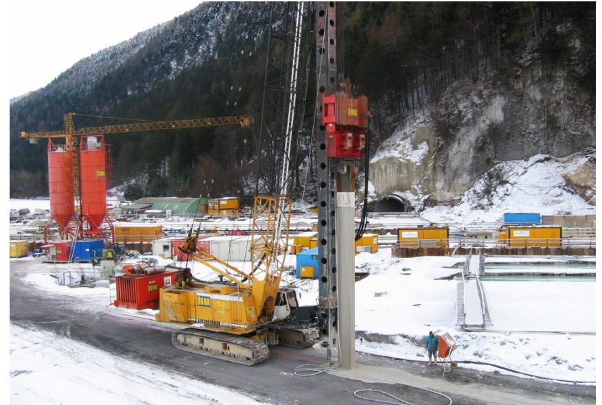
2005: Brenner Railway – Cut and Cover Tunnel
