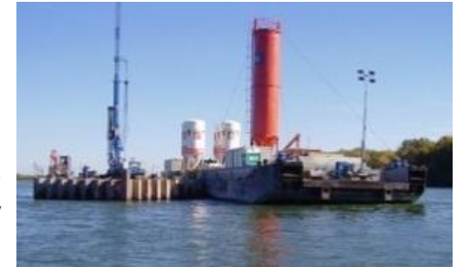
2007: ÖBB Railway Bridge
